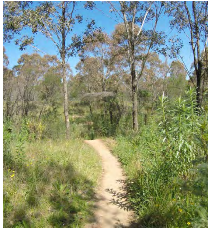
A footpad track using natural soil is the preferred track construction technique for cost effectiveness and a natural look and feel
